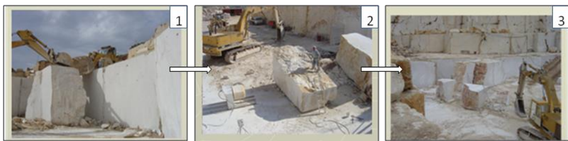
Fig. 2. Illustration of the three steps of the excavation of “Perlato di Sicilia”.
